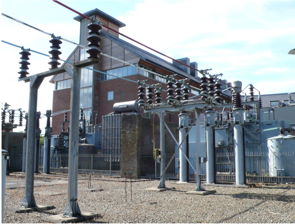
figure 01 NEDL primary substation
